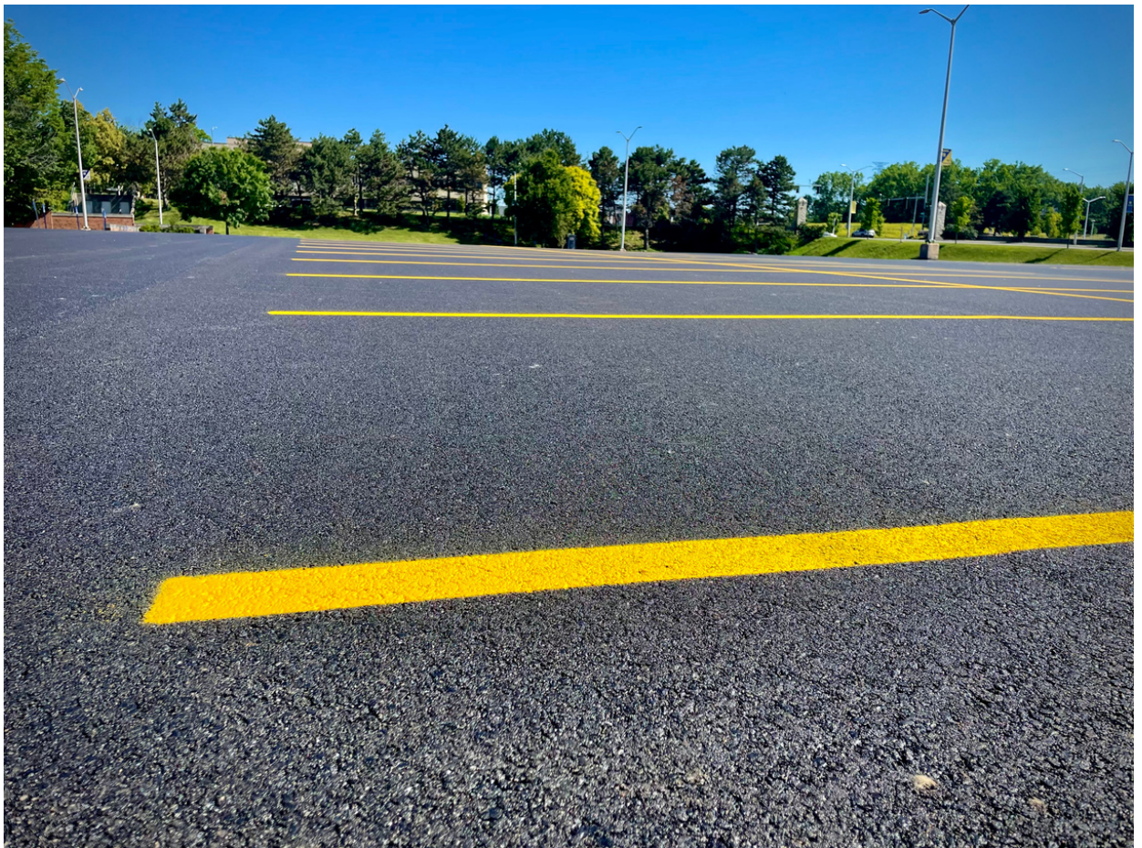
Area 1N - Newly renovated surface parking lot.
